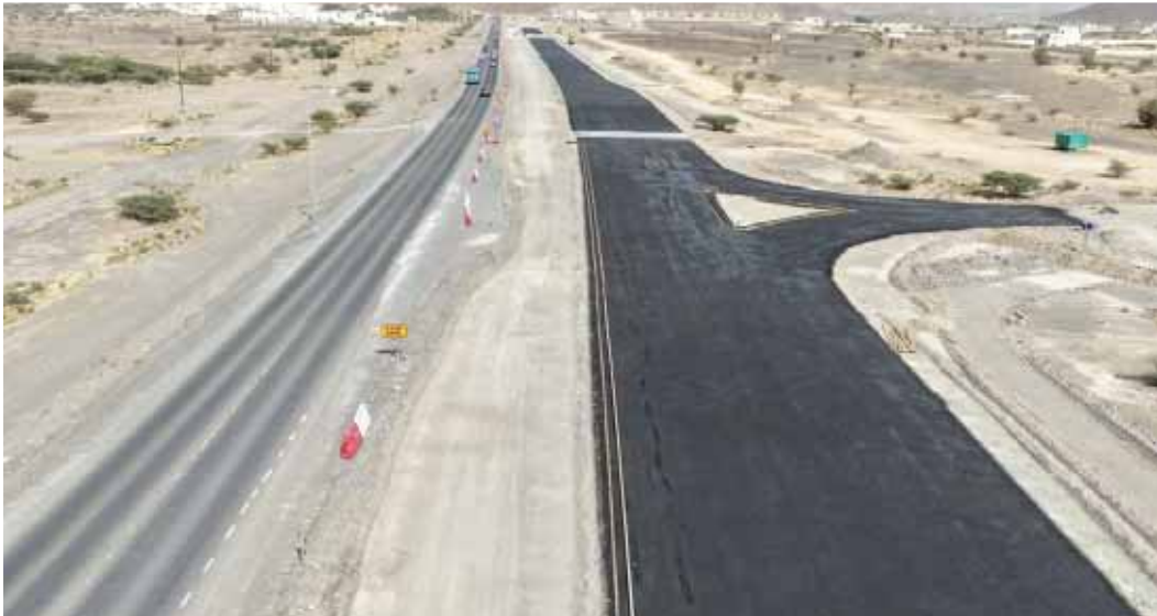
ROAD NETWORK: Asphalt road maintenance works across the governorate continue with an approximate cost of OMR6,004,000, covering a total length of 1,244 kilometres. - ONA
