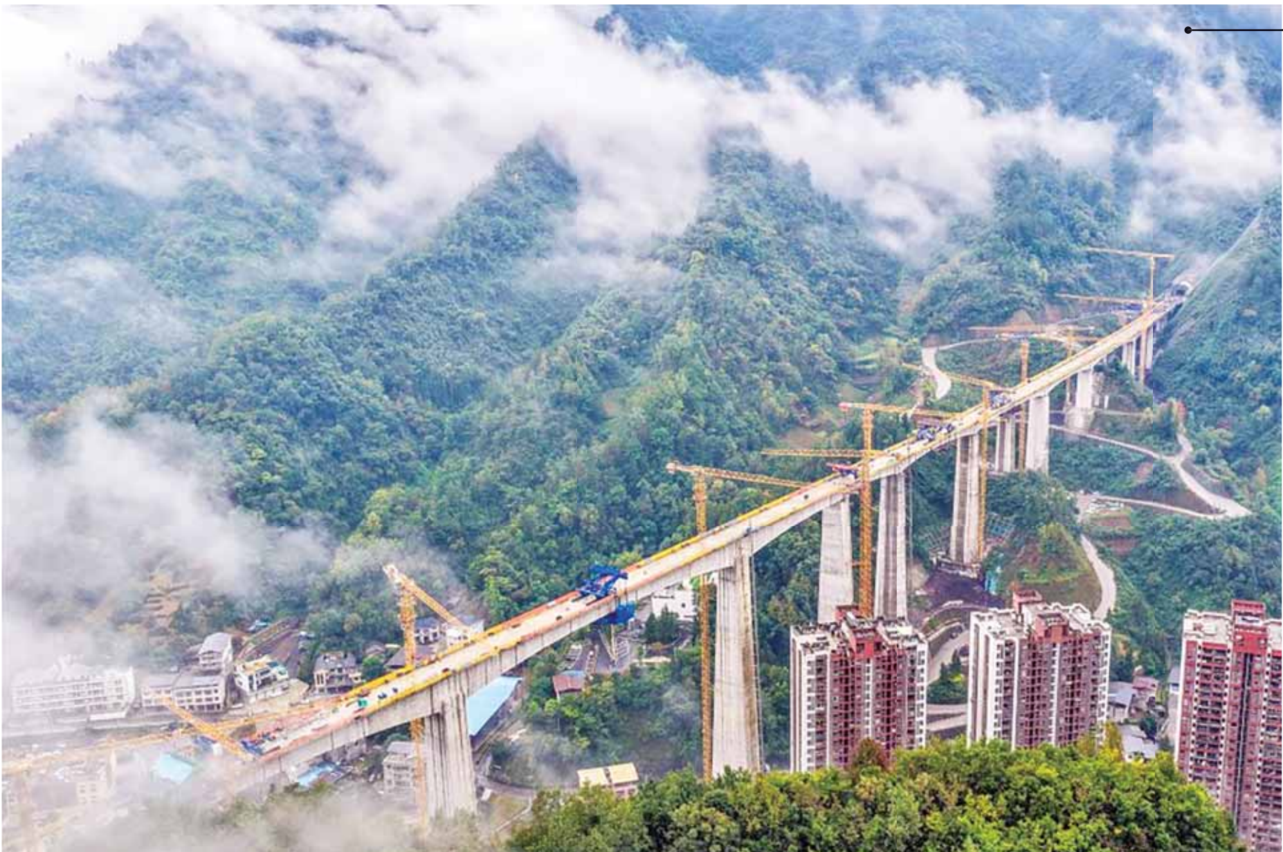
CONSTRUCTION SITE OF THE MIAOJIALIANG GRAND BRIDGE IN CHINA: An aerial drone photo shows the construction site of the Miaojialiang grand bridge in southwest China's Chongqing Municipality. Located in Chengkou County of Chongqing, the 941.6-metre-long Miaojialiang grand bridge, a key project along the Xi'an-Chongqing high-speed railway, was successfully closed here. — Xinhua
